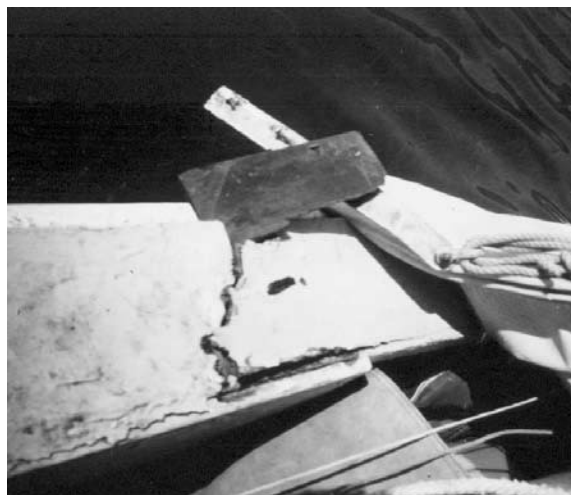
Damage due to chainplate failure
